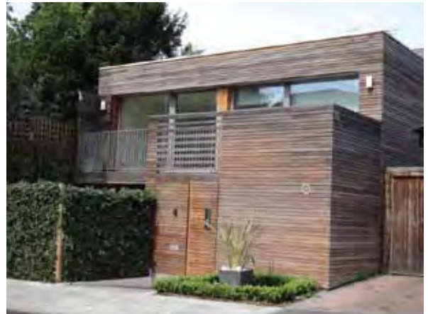
Figure 4: The Camden Passivhaus by Bere Architects, focus of a TSB project. Courtesy of Olivia Guerra-Santin
