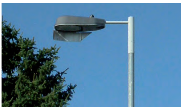
Figure 3: Luminaire fitted with a screen to limit spill light reaching a nearby garden
