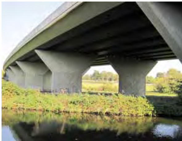
Figure 1: Concrete viaduct supporting the M25 motorway at King's Langley, Hertfordshire
