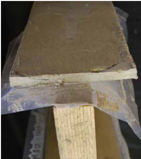
Figure 2: Thin structural concrete topping on a timber beam
