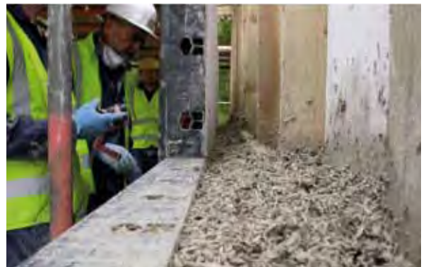
Figure 1: Casting a hemp-lime wall
