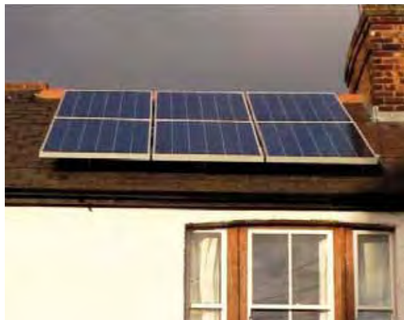
Figure 1: Typical retrofitted BAPV array
