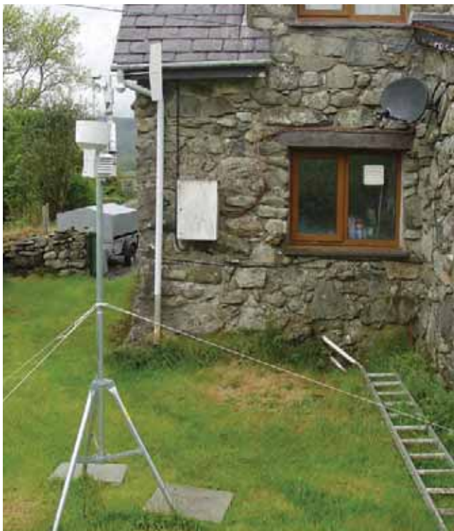
Figure 2: Monitoring the hygrothermal performance of upgraded thick, stone walls in the harsh climate of North Wales. Courtesy of Shiyu Jiang
