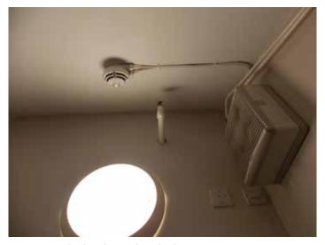
Figure 6: Poorly placed optical smoke detector
