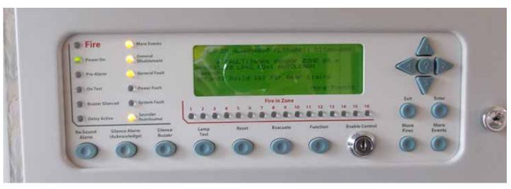
Figure 15: Example of panel in fault and isolate condition
