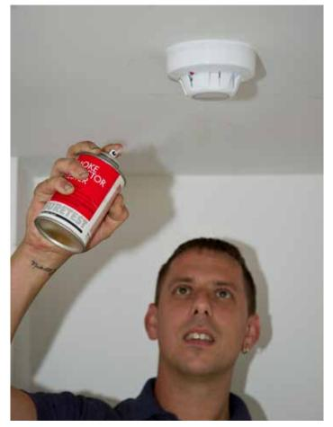
Figure 11 Weekly test of fire detection system
