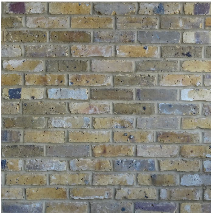
Figure 1: Example of internal wall (brick) used for gathering measurements
