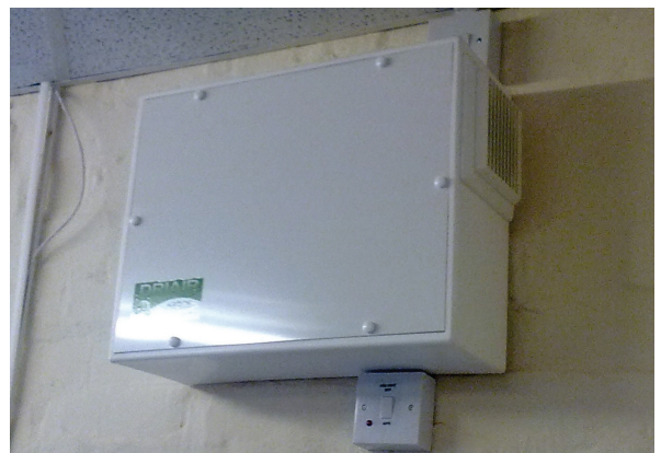
Figure 2: Wall-mounted positive ventilation system
