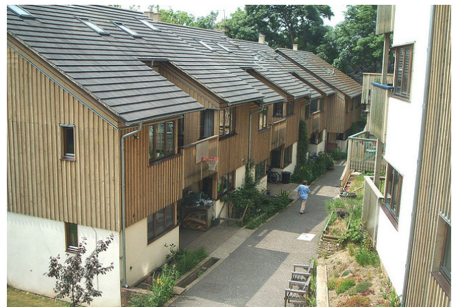
Figure 2: Springhill Cohousing, Stroud, by Architype Architects. Timber-framed houses insulated with Warmcel, clad in local timber (image © Stephen Hill, C20 futureplanners)
