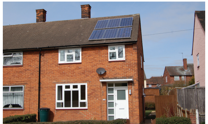
Figure 1: Refurbished dwelling (House 18)
