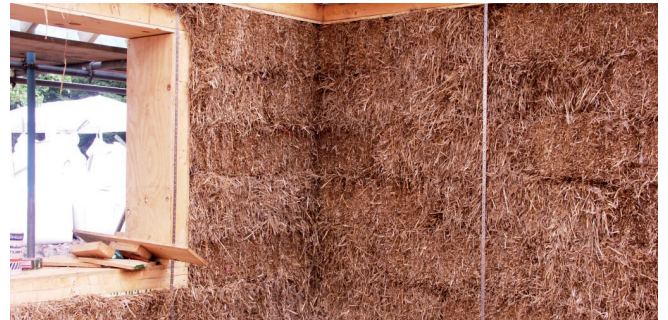
Strawbale wall construction
