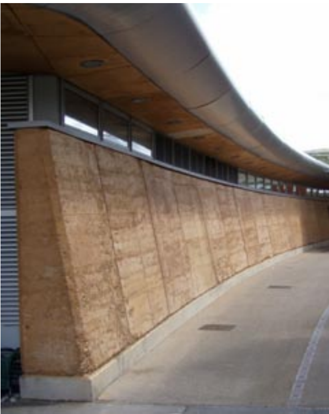
(Grimshaw architects; In Situ Rammed Earth; 1999)
