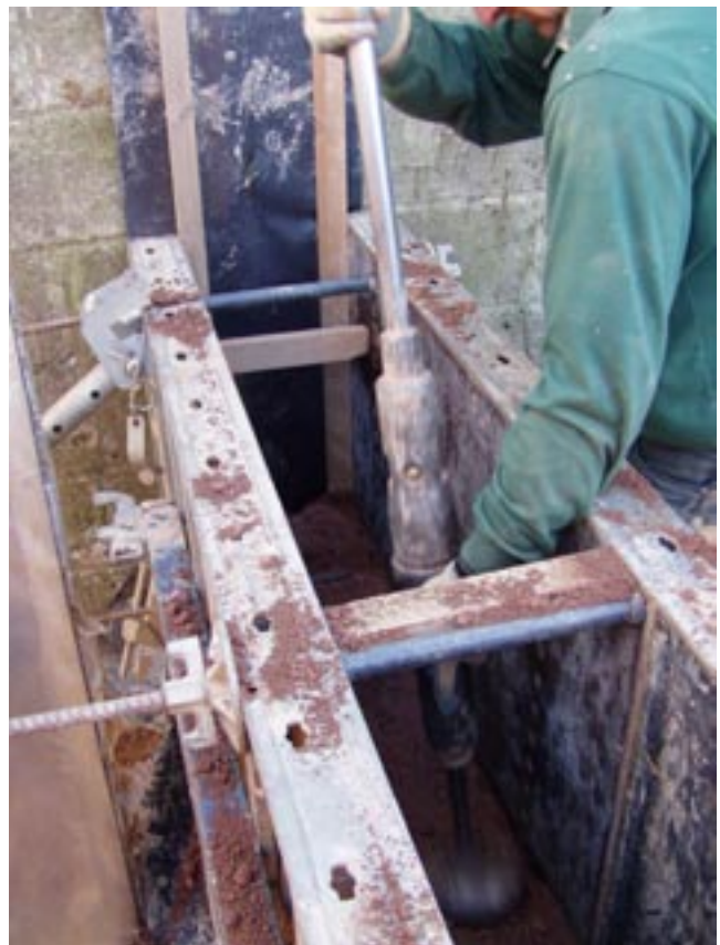
Figure 2 Construction of a rammed earth wall
