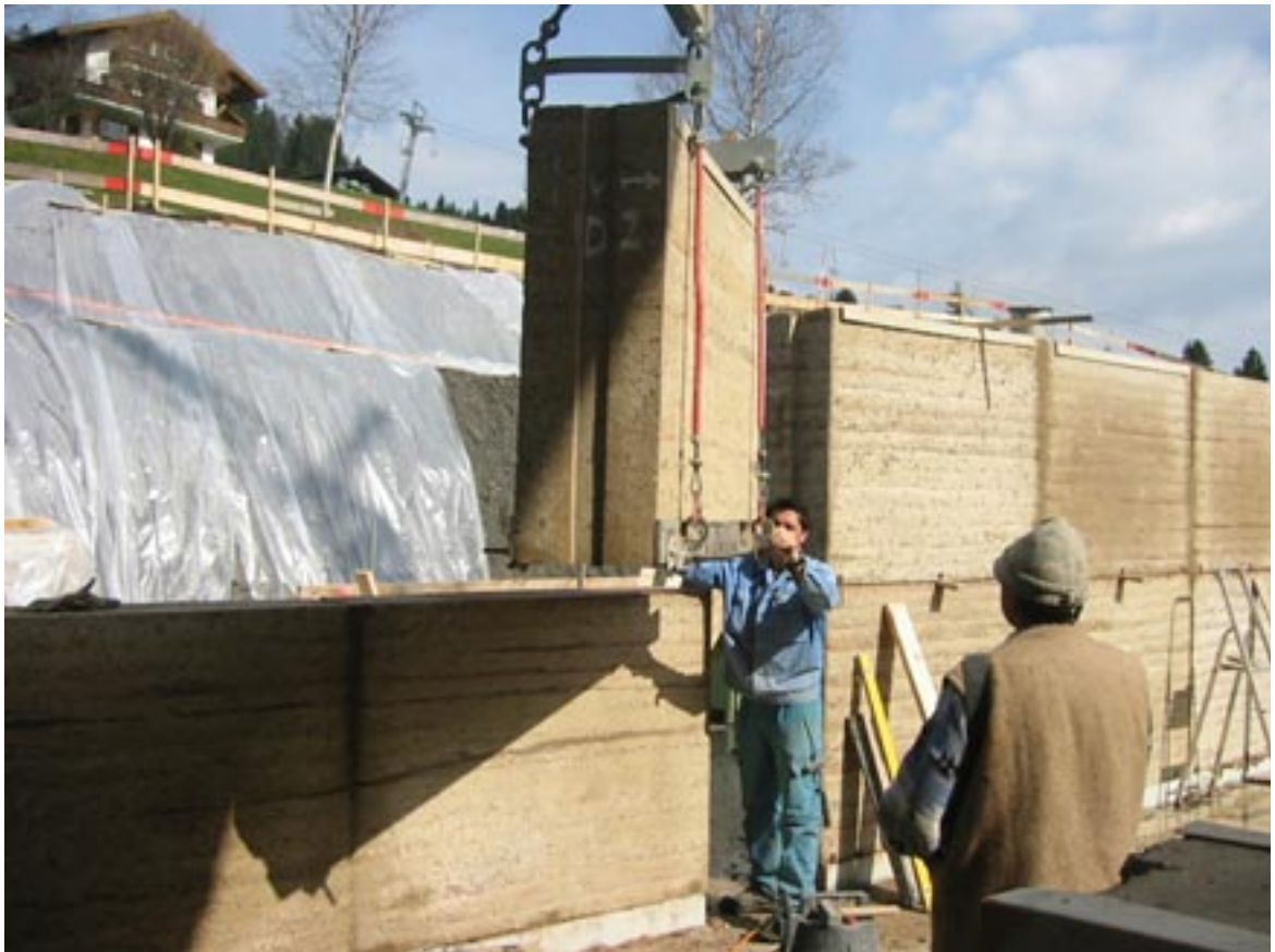
Figure 27 Prefabricated rammed earth walls
