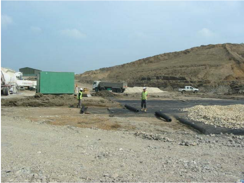
Photo 7 Placement of reinforced platform in layers
