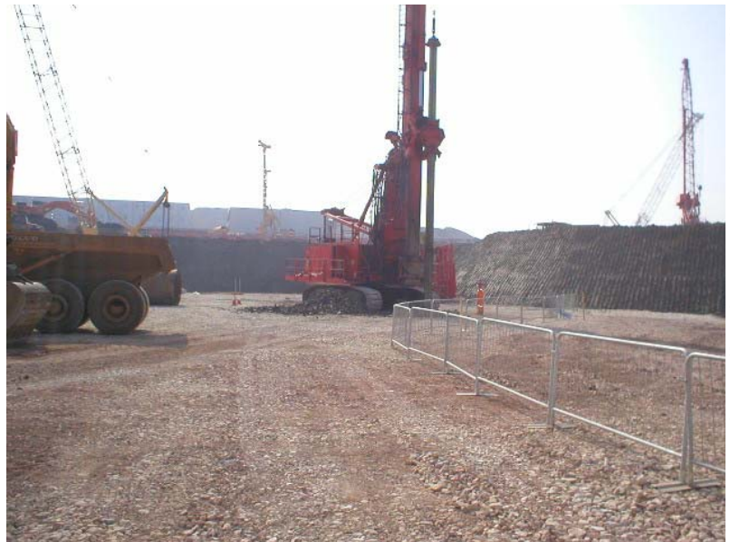
Photo 8 Good control during platform installation – unfinished areas fenced off to prevent access
