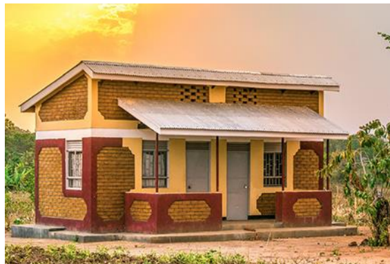
Meeting the huge global housing demand requires affordable and sustainable building materials. (Image courtesy of HYT Uganda)
