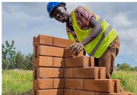
Cement-stabilised earth blocks have lower financial and environmental costs than fired clay bricks. (Image courtesy of HYT Uganda)
